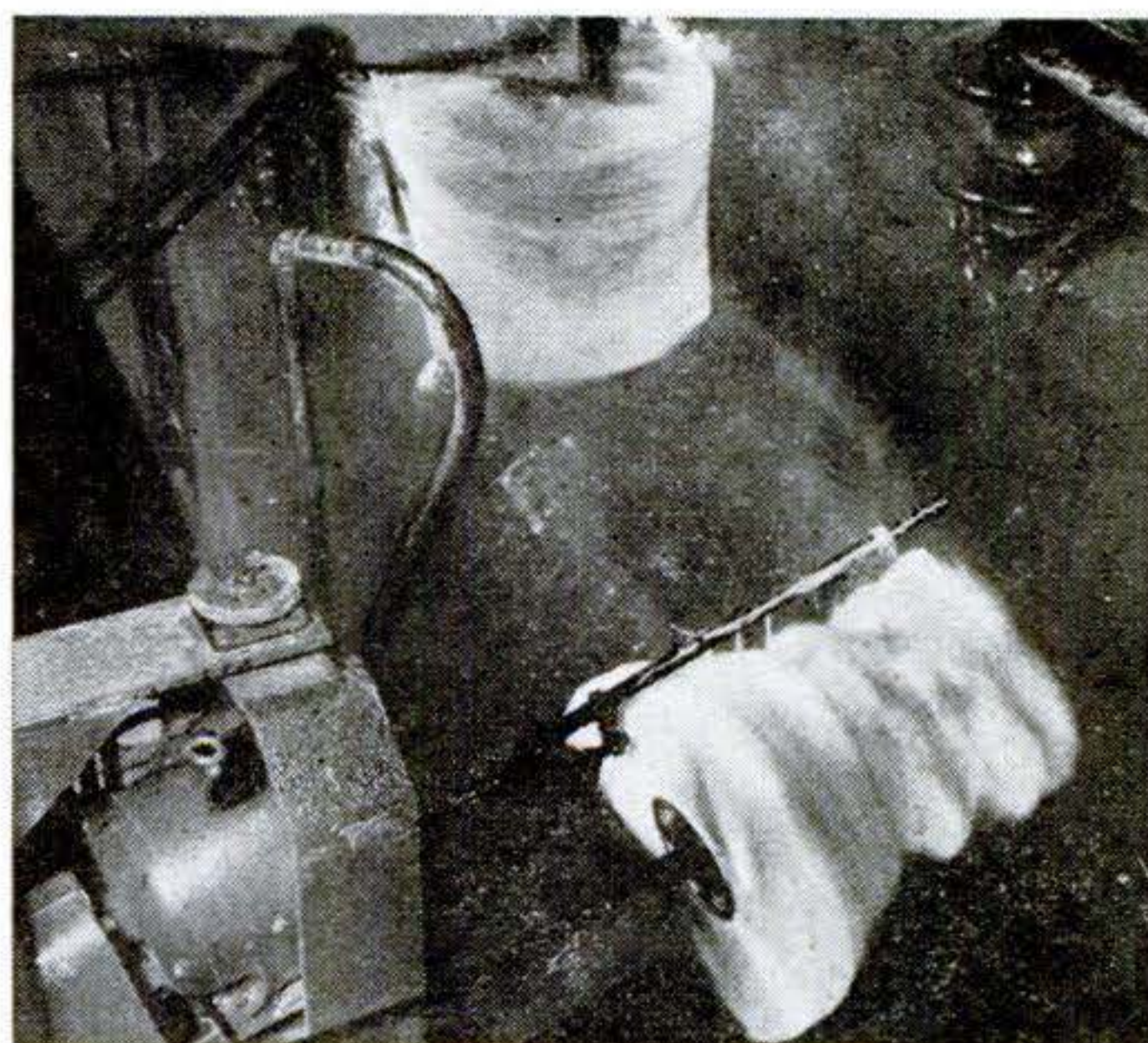
6. On top , two brushes to a side share vertical and horizontal surfaces. There are two complete brush installations; first set cleans, second set polishes while engine is rinsed.
